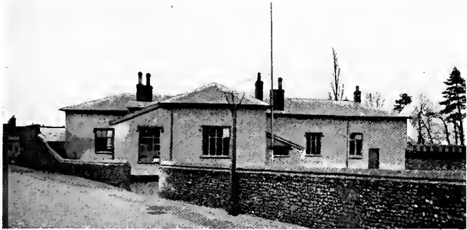
ONCE CORN HALL, NOW COUNCIL SCHOOL. Built about a hundred years ago. Still in sound condition and quite dry.
